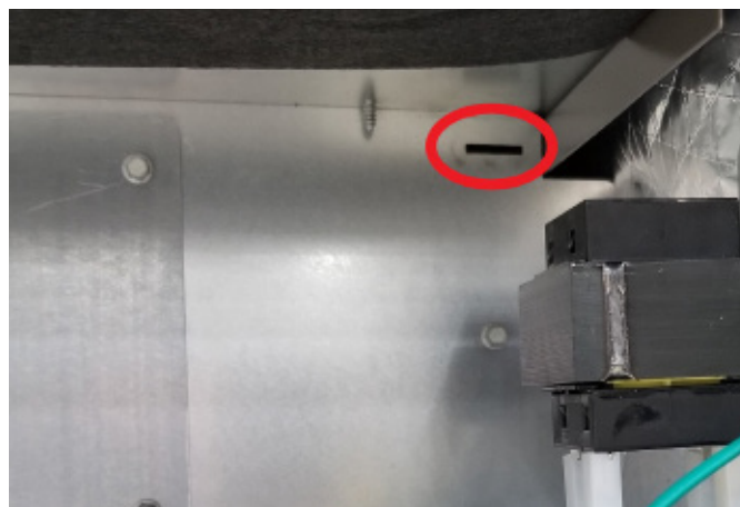
FIGURE 18. Notch for Control Panel Relocation
