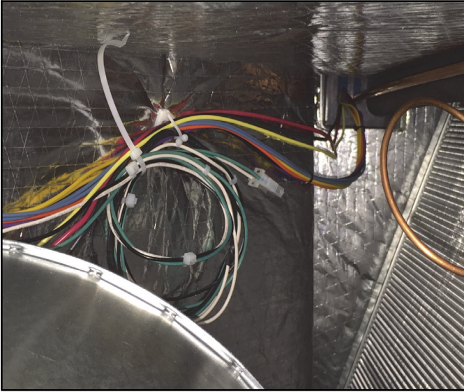
Figure 8. PCO Wire Harness in Wire-Tie
