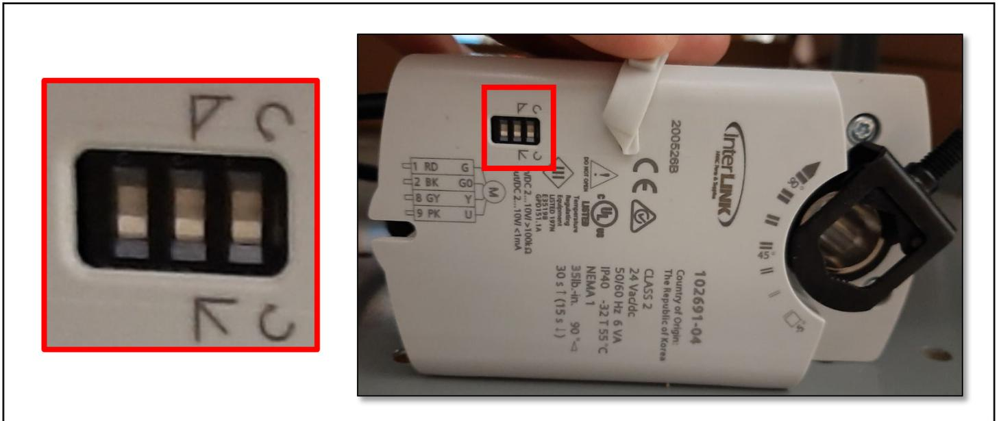
Modulating Actuator DIP Switches with Correct Settings
