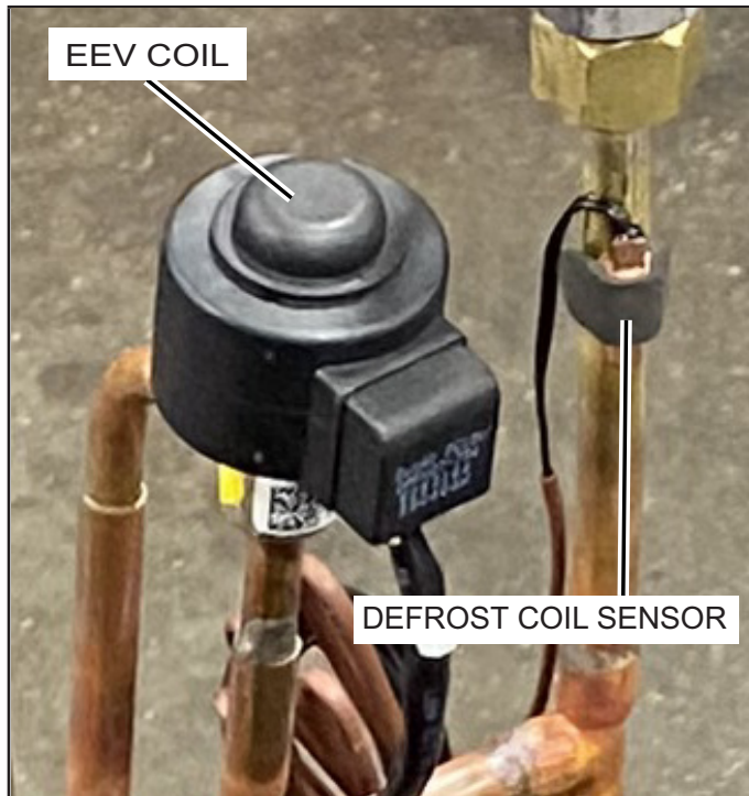
FIGURE 21. Defrost Coil Sensor Location
