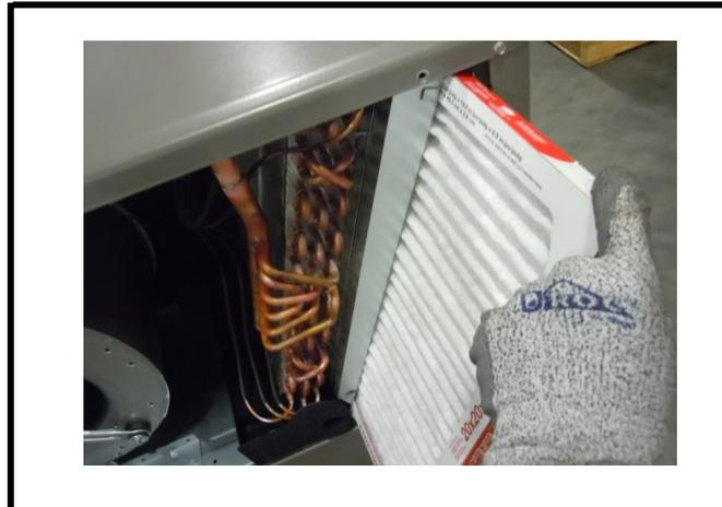
Fig. 10: Inserting Filter into Rack
