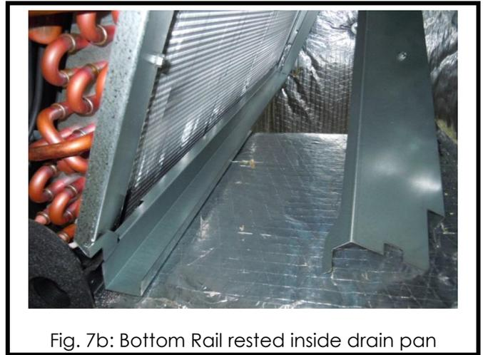
Fig. 7b: Bottom Rail rested inside drain pan
