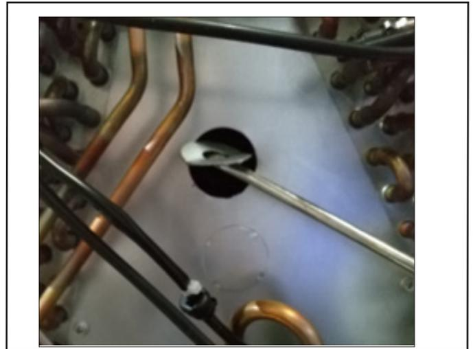
**Figure 7. Remove T1 Sensor Knockout**
