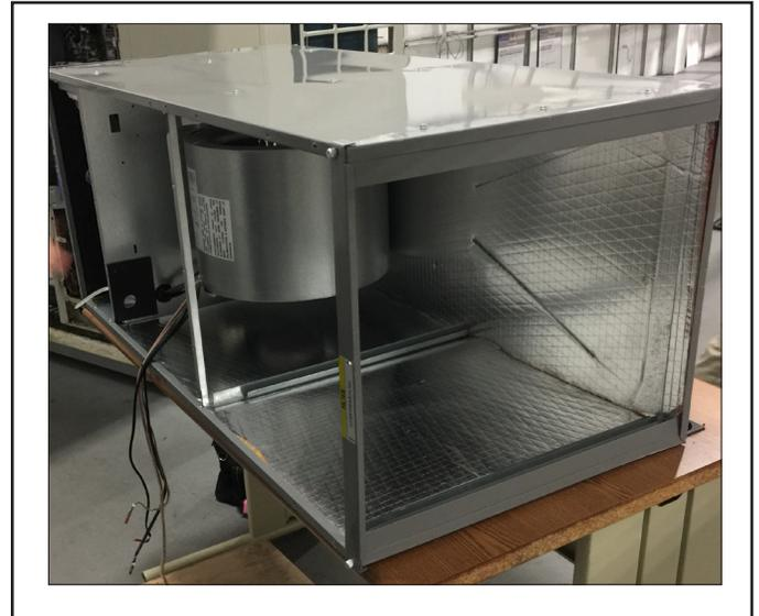
**Figure 8. Position Cabinet in Horizontal Left Orientation**
