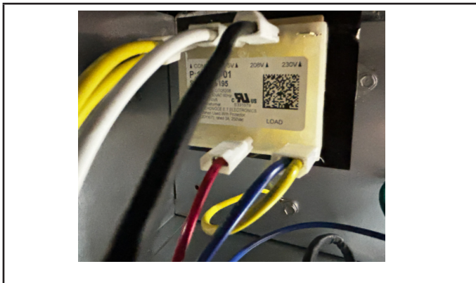
FIGURE 23. Converting Unit from 230VAC to 208VAC
